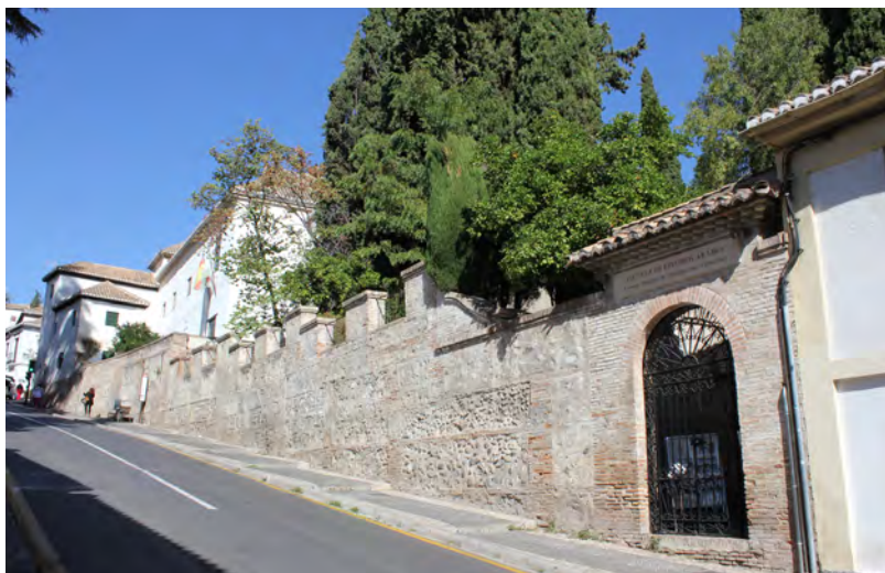
EEA - The entrance
